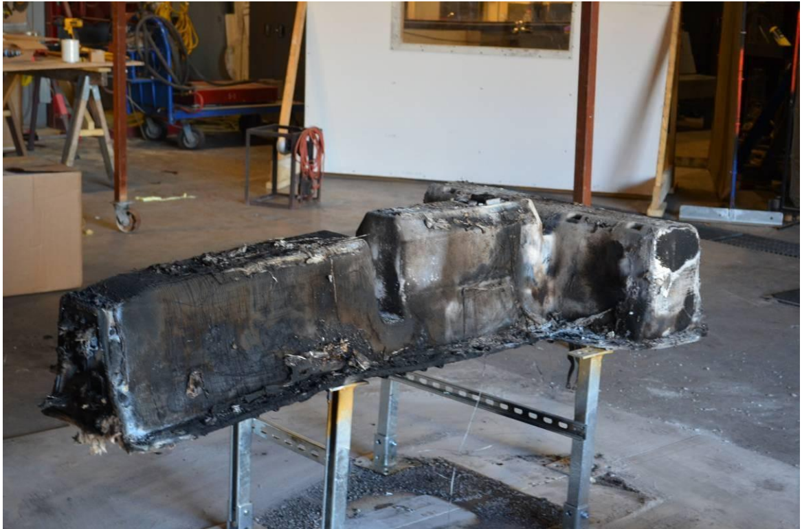
Figure A-13. Post-Test View of Battery.
